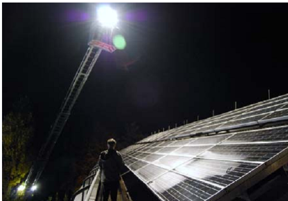
Fig. 1: Situation at the PV generator of sub-plant West of the PV test plant of BFH-TI under illumination by two floodlights of 1 kW on Oct. 27 th , 2010 by the fire brigade of the town of Burgdorf (minimum distance 7 m).
