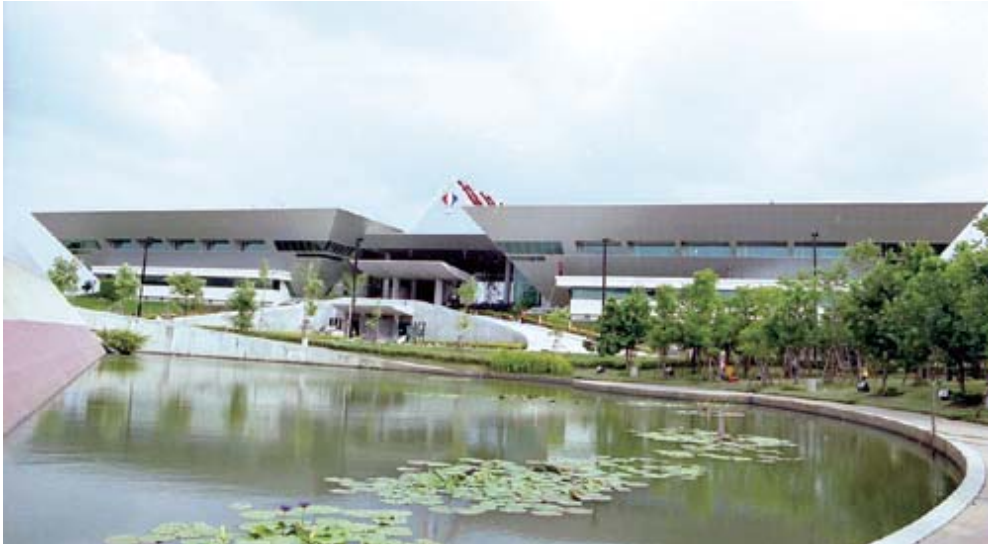
Fig. 33: Just-constructed new laboratory building (May 2005)
