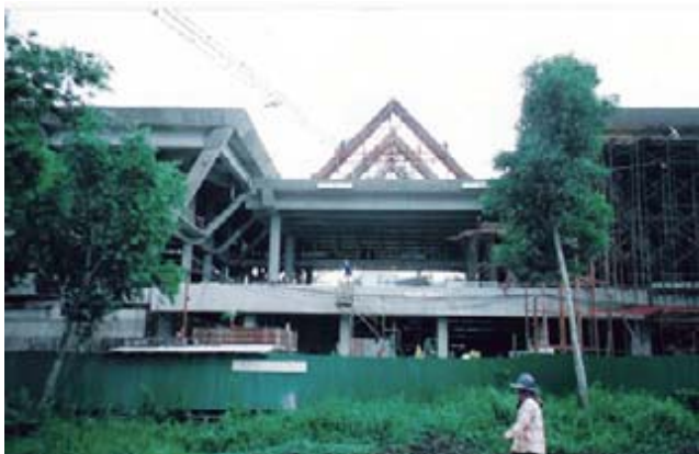
Fig. 17: Entrance building with open-air structure
