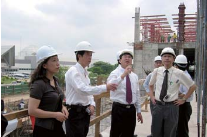
Fig. 18: Survey group receiving briefing on the new laboratory building during construction. Mr. Somsak Charkkian of NIMT (in the middle) giving the explanation.
