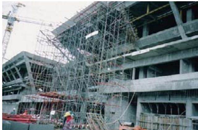
Fig. 16: Second laboratory building. Construction of the overhang to prevent strong sunlight was quite a difficult work.
