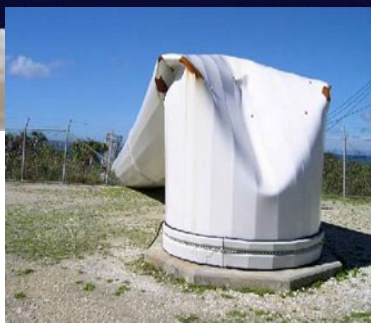
Tower buckled by Typhoon (Happened on 2003/9/11 at Miyako island in south of Kyusyu, JP)
