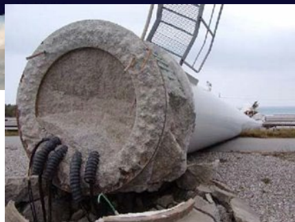
Tower buckled by Typhoon (Happened on 2003/9/11 at Miyako island in south of Kyusyu, JP)
