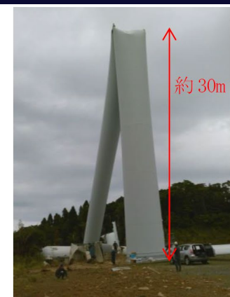
Broken Blades Typhoon (Happened on 2016/9/20 at Kimotsuki, Kagoshima, Kyusyu JP)
