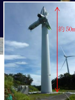
Broken Blades Typhoon (Happened on 2016/9/20 at Kimotsuki, Kagoshima, Kyusyu JP)
