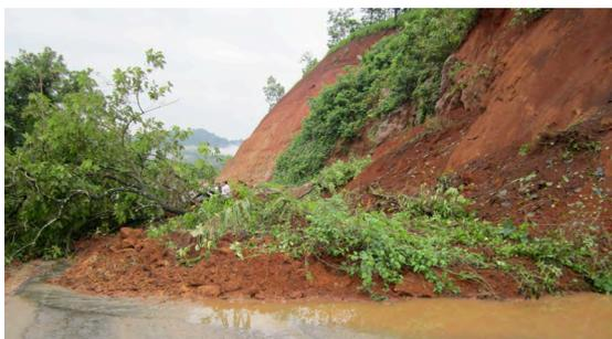
**Fig. 2.** Landslide triggered after overnight rainfall blocked NH-40, Ri-Bhoi district, Meghalaya
