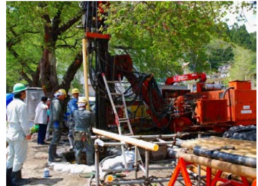
Drilling at Otsuchi-town, Iwate.
