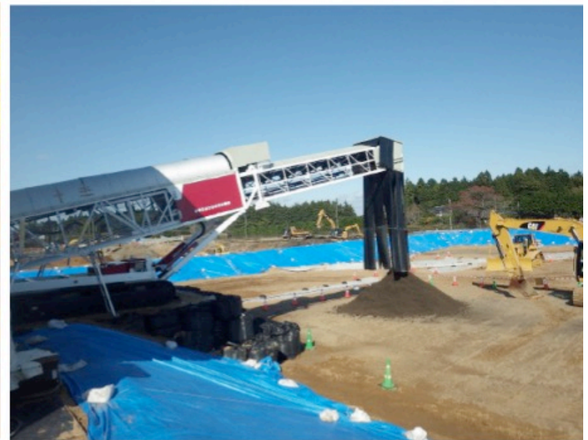
Soil Storage Facility (First period in Okuma) (Planned storage volume approx. 210,000m 3 )
