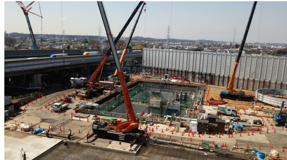
Construction site for Tokyo Outer Ring Road
